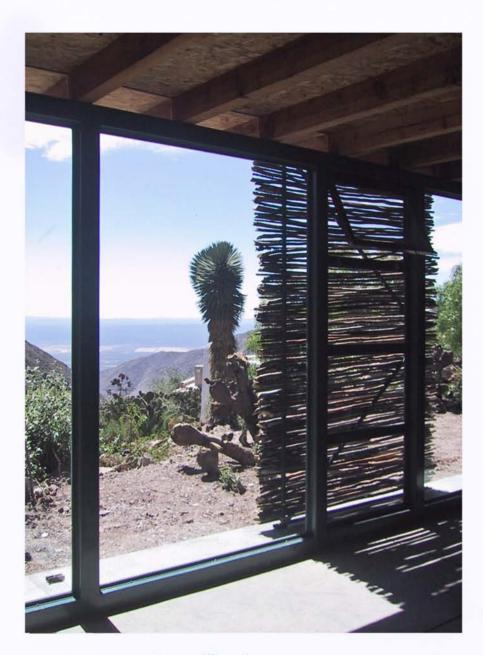
are simple and pragmatic. There is a difference between a simple appearance and simplicity in the production process. The latter can even be a guide to constructive expression, as here in the use of herding staves for the sliding panels that serve as sunscreens.
